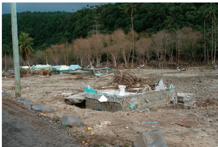
Demolished buildings post tsunami
